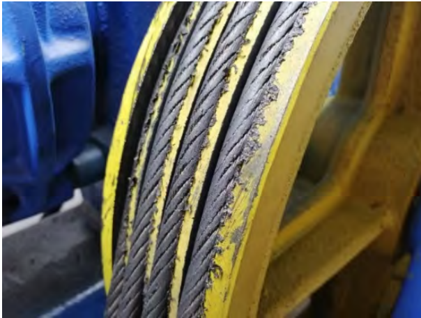
Picture 3. Worn pulley and lack of rope tension adjustment
