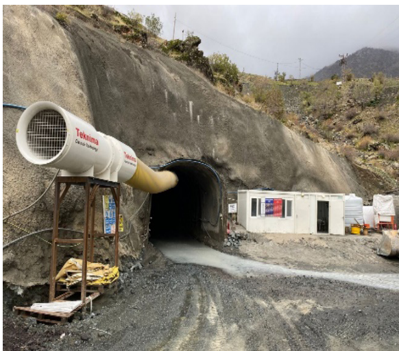
Figure 4. Mine main entrance gallery and ventilation system
