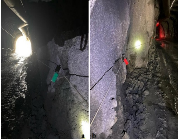
Figure 14. Applications a lifeline using green reflection in the direction of exit from the mine [a] and red reflection in the danger zone [b]
